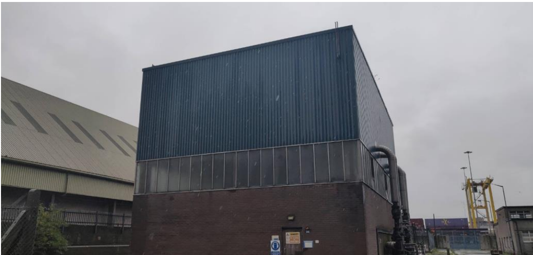
Figure 5.2: Existing buildings located within the proposed development site
