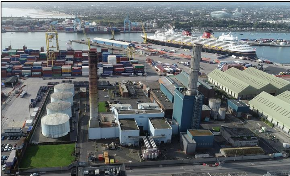
Figure 5.1: Existing North Wall Power Plant facility (drone footage, looking south)
